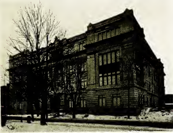
New High School Building North Washington Street (Under Construction)
